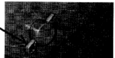
CORRECT METHOD OF RETAINING ROCKER PAD PIN WITH COTTER PIN
