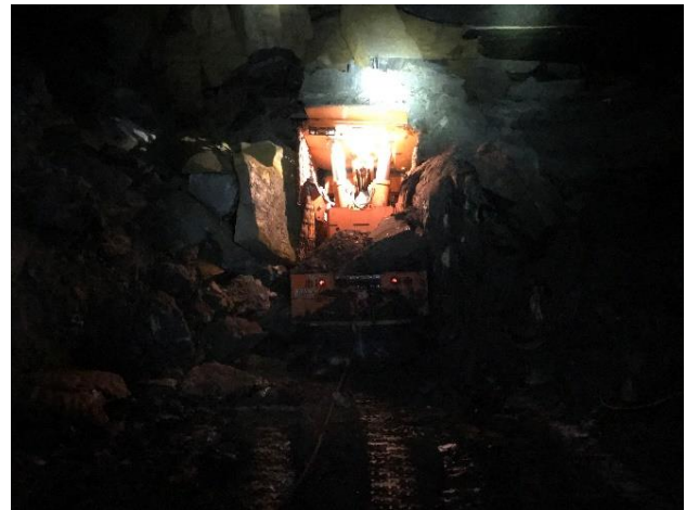
Figure 9. Mobile Roof Support Working
