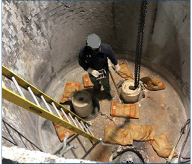
Typical refractory re-lining area within ladle.
