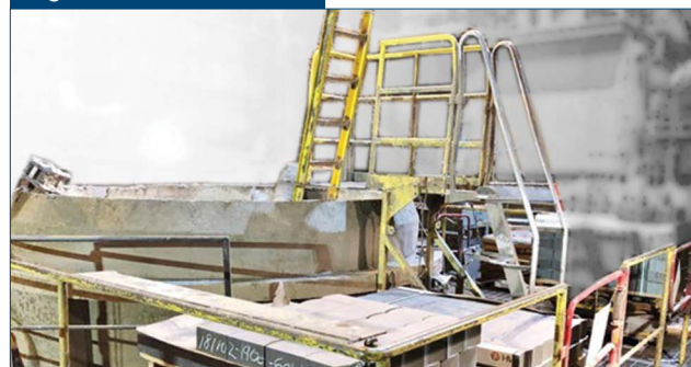
Typical work deck platform area.
