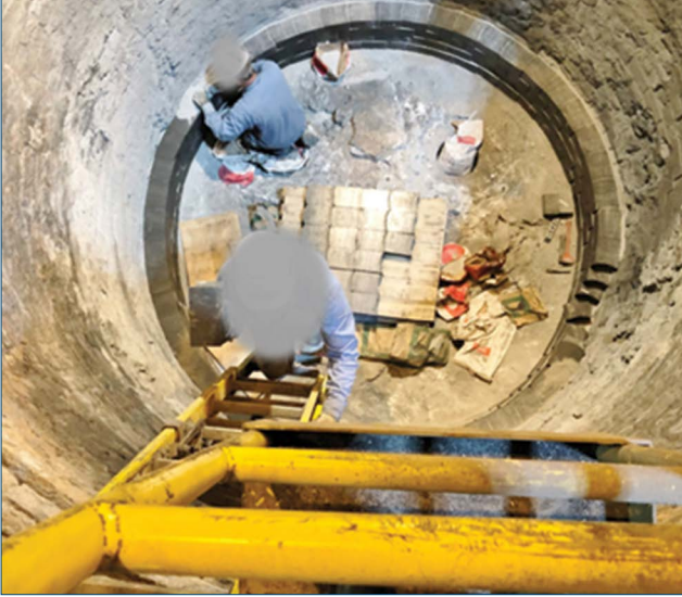
Typical refractory re-lining area within ladle.
