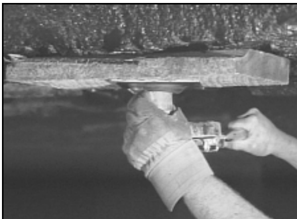
Checking Bolt Torque With Torque Wrench
